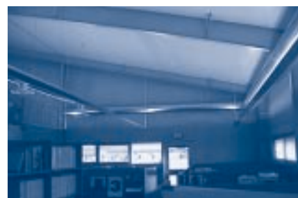
The metal panel walls in the office building create a clean, comfortable workspace and eliminate the need for interior finishes. Employees need not strain their eyes due to both abundant indirect lighting and daylighting.
